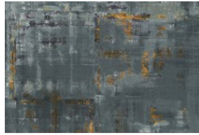
8994 Paint Scrape Steel.jpg
